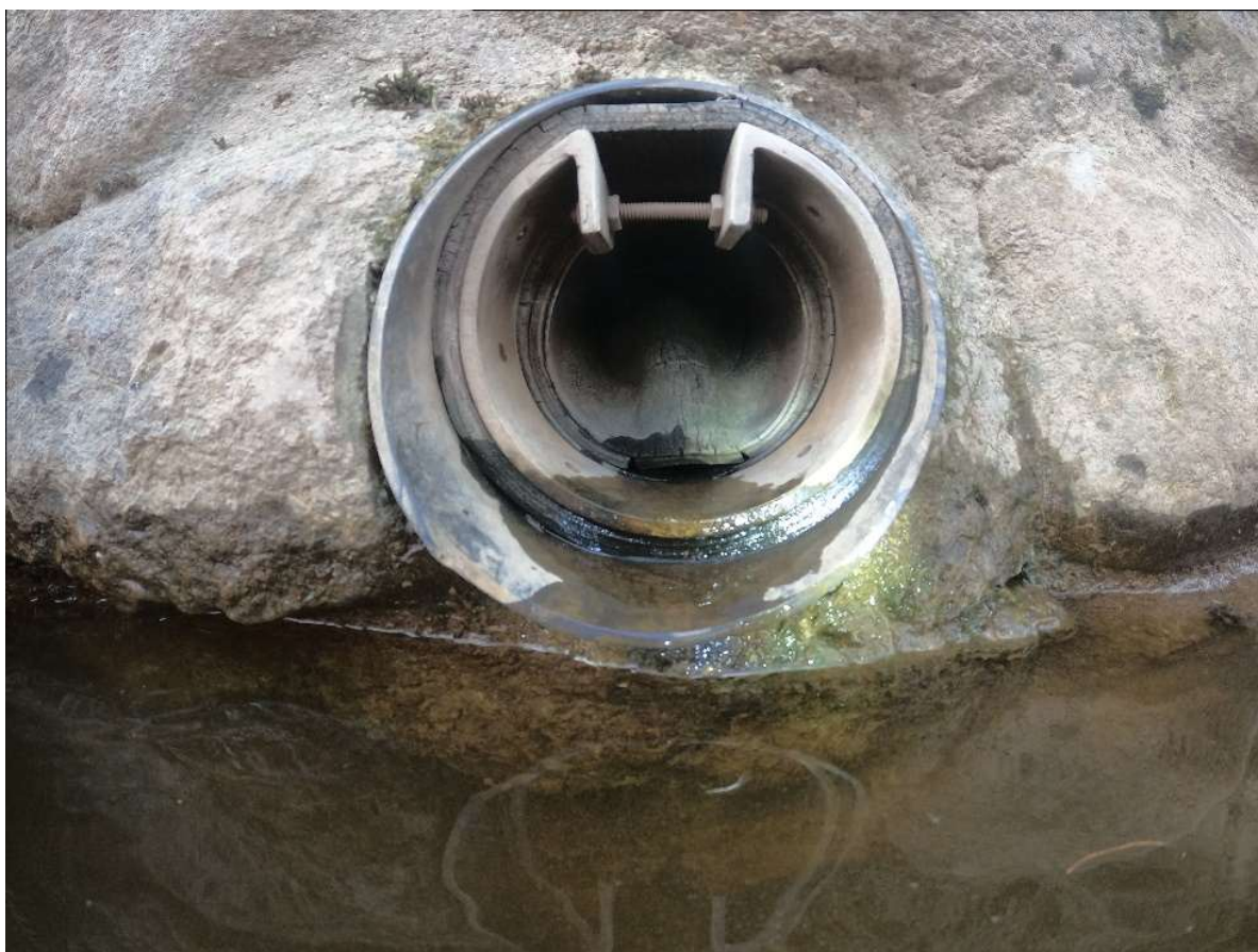
Figure 1-10: NRV placed on a pre-existing outfall in Graiguenamanagh.
