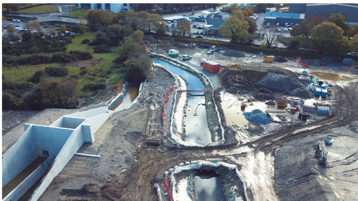
Figure 1-3: Example River diversion (on right) with access crossing to allow structure construction in watercourse (left)
