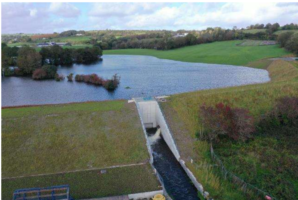
Figure 1-4: Example storage area with flow control structure in flood conditions (Source: https://www.wardandburke.com/project/river-feagle-clonakilty-certified-drainage-scheme/ )
