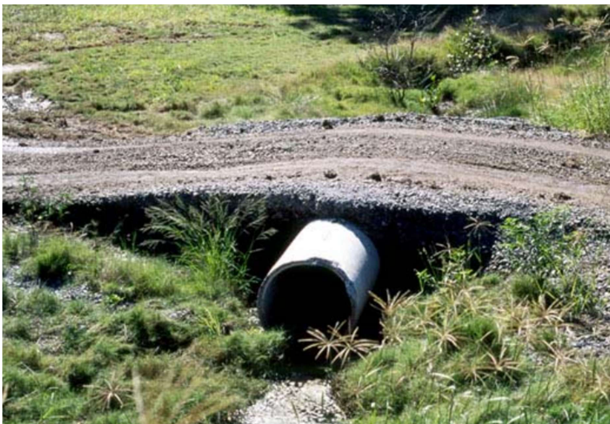
Figure 1-5: Example temporary river crossing (Source: https://www.austieca.com.au/documents/item/319 )
