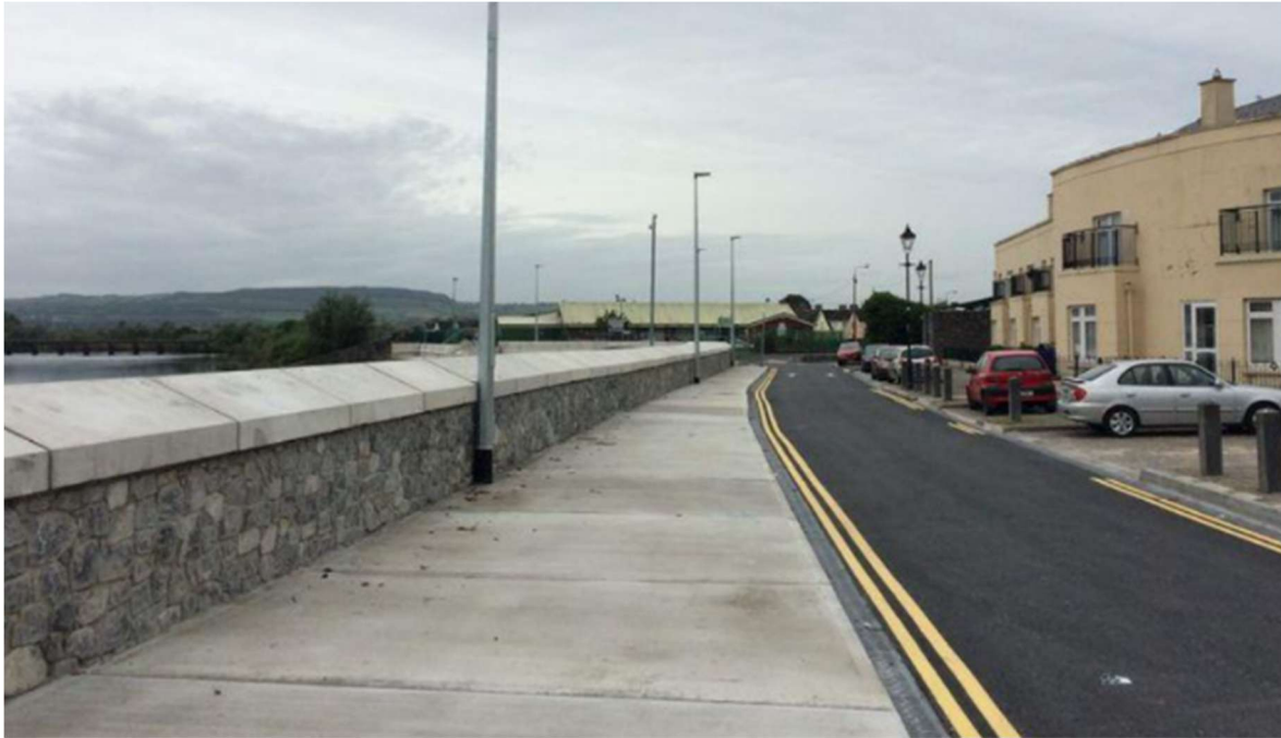
Figure 1-7: Example wall construction including stone facing.
